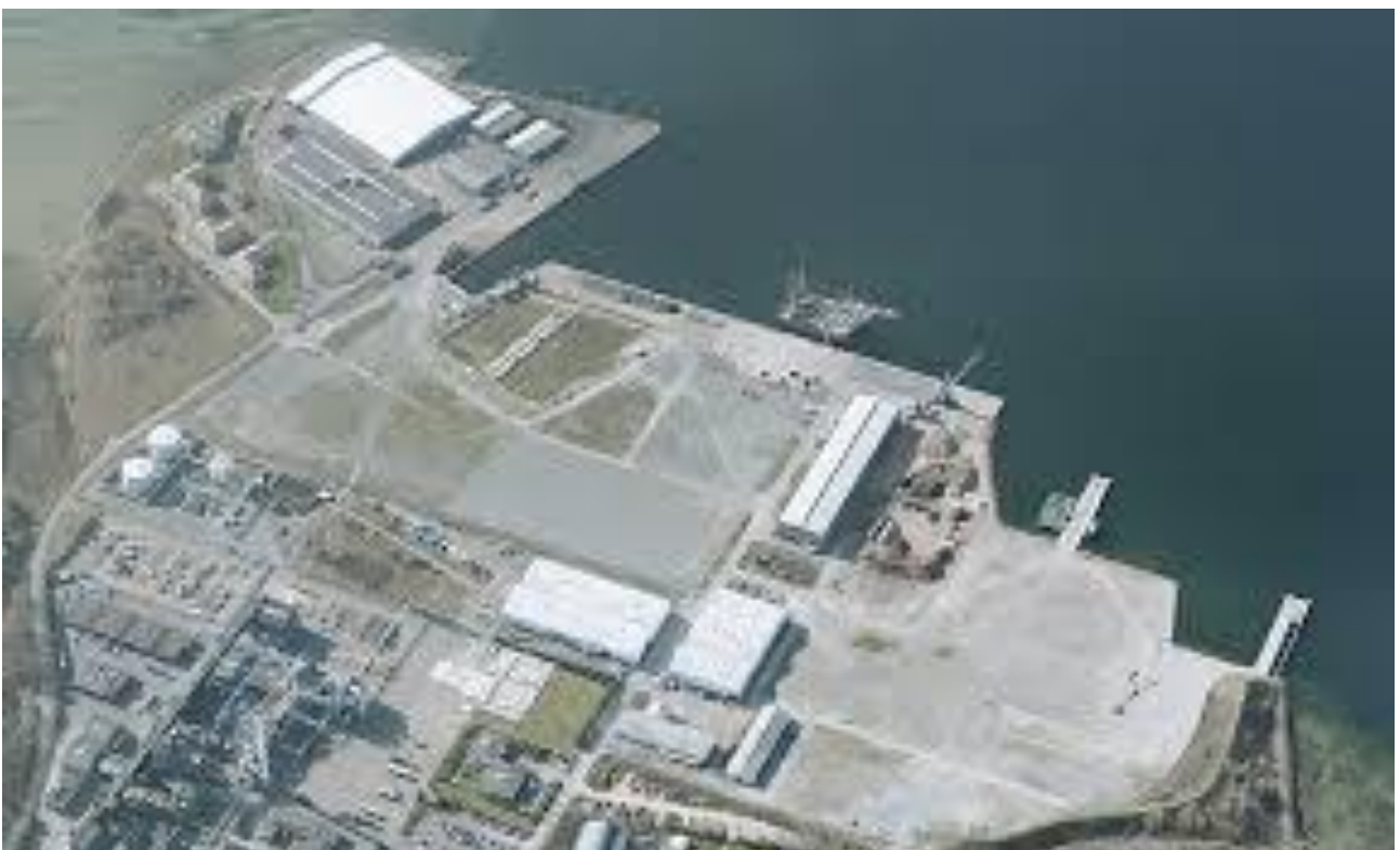
Above: An aerial photo of the land of the planned plant in Nyborg, Denmark
